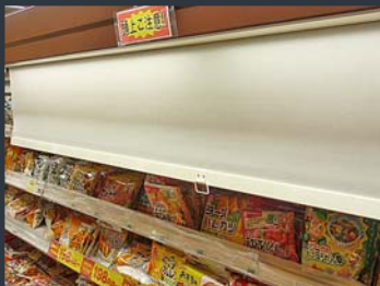
Night cover installation to maintain cooling at night
